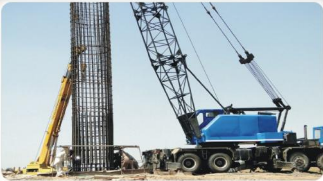
Cage Lower in Bored Pile using Heavy Crane
