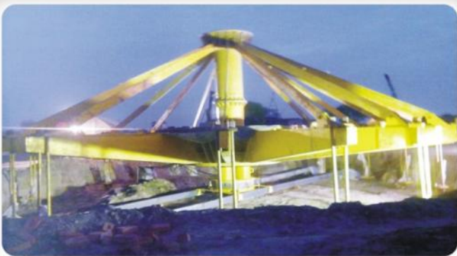
Pile Load Test Activity using Anchorage System Method
