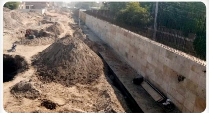
Earthwork activity on Retaining Wall at Madni Chowk Flyover, Multan.
