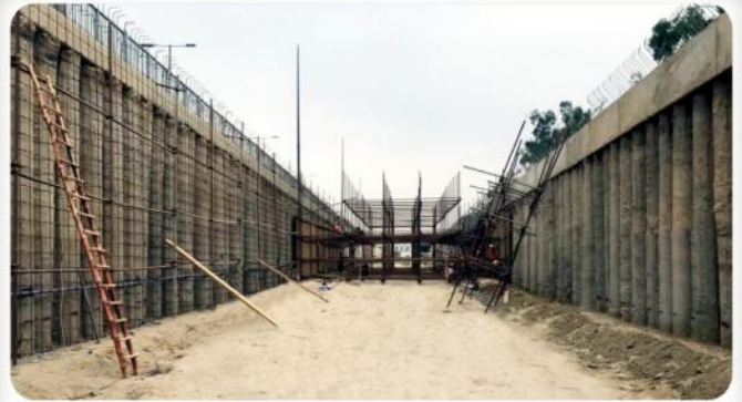
Construction of Underpass Face Walls at Ghulab Devi Hospital Underpass, LHR.
