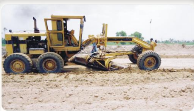
Leveling of Embankment Activity using Motor Grader
