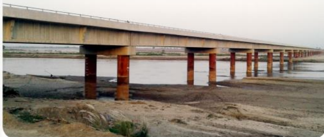
Sultan Bahoo Bridge over River Chenab Pkg-I-Main Bridge
