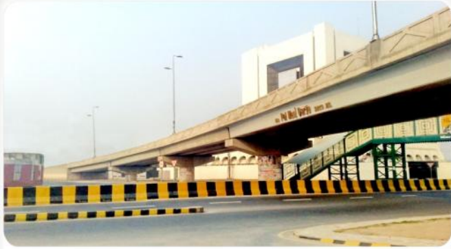
Pul Moaj Darya Flyover Along with Pedestrian Bridge For Inner Ring Road, Multan Pkg-III.
