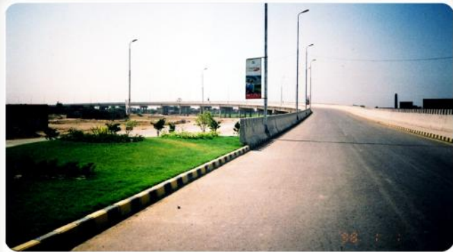
Overhead Bridge at Railway X-ing for G-Magnolia Park Housing Scheme, Gujranwala
