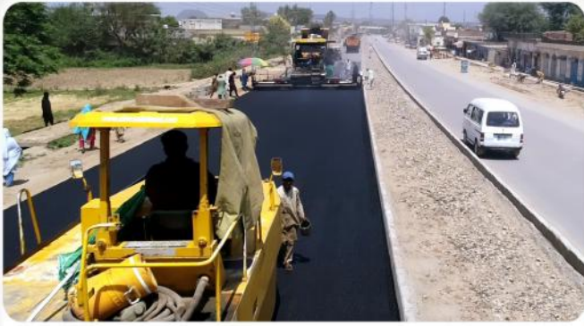
Asphaltic Concrete Activity at Dina Mangla Road, Dist. Jhelum.
