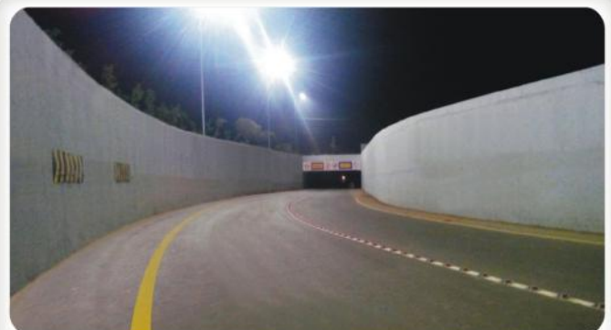
Under Pass at Bhaini Road For Lahore Ring Road Project
