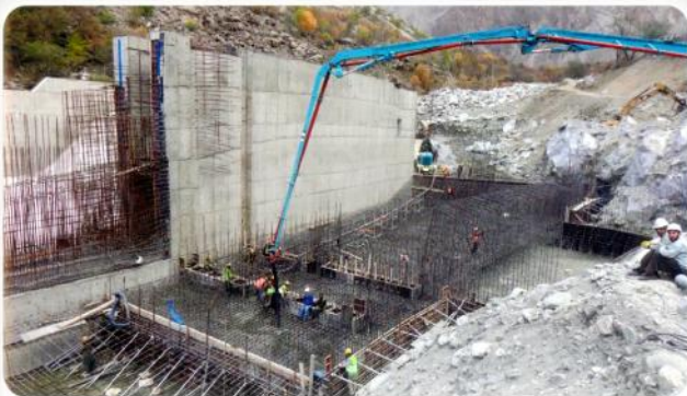
Stilling Basin Concrete
