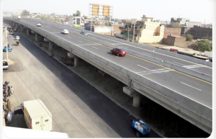
A side view of Completed Bridge Structure Shaheen Chowk Flyover, Gujrat.
