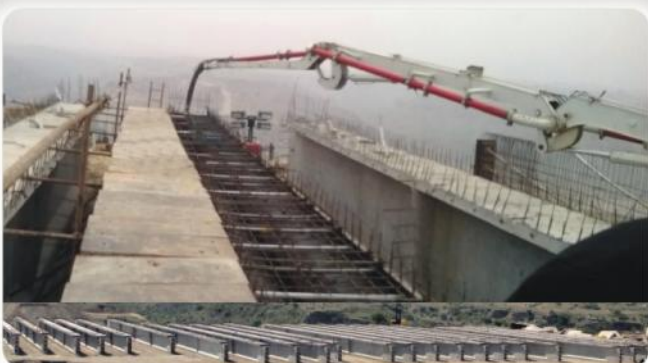
Concrete Pouring in Girder through Concrete Pump
