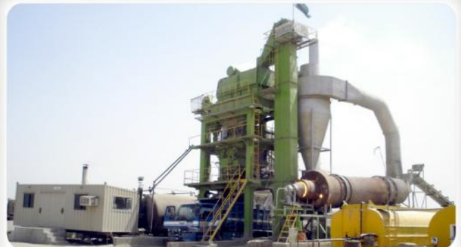
Asphalt Plant Shinseang (SPECO) (80/100 Ton/Hr) Working at Dina,
