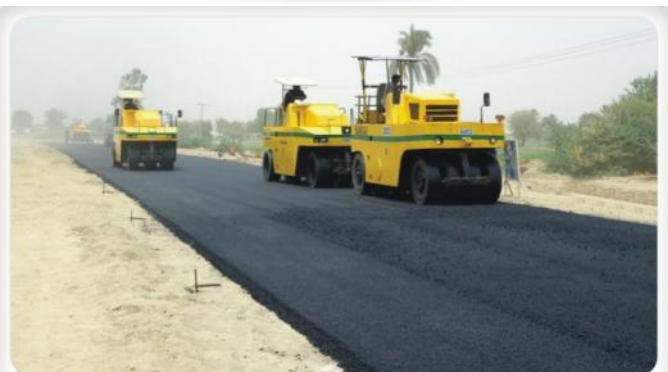
Compaction of Asphaltic Concrete Using PTRs
