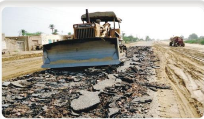
Existing Road Dismantling Activity using Heavy Bulldozer
