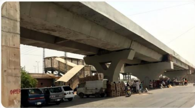
A side view of Completed Structure at Madni Chowk Flyover, Multan.
