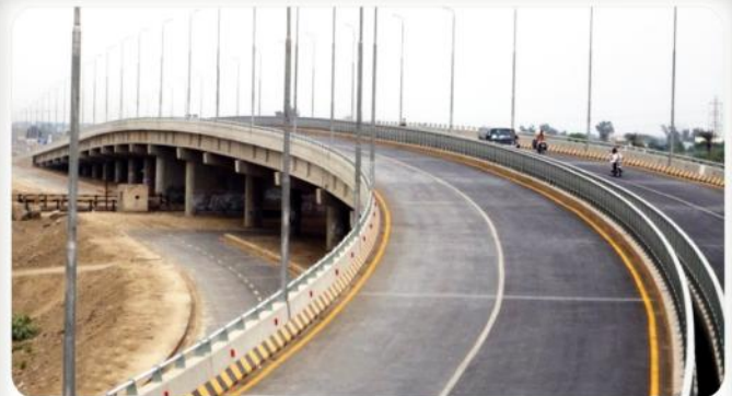
Overhead Bridge (DCW) at Railway X-ing, Bahawalpur.
