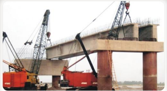
Launching of Concrete Girder using Heavy Cranes
