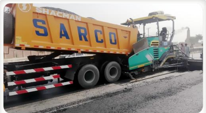
Asphaltic Concrete Laying Activity Using Vogele 1900-2 Asphalt Paver Machine
