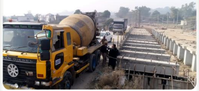
Concrete Activity on Vented Causeway at Dina Mangla Road, Dist. Jhelum.
