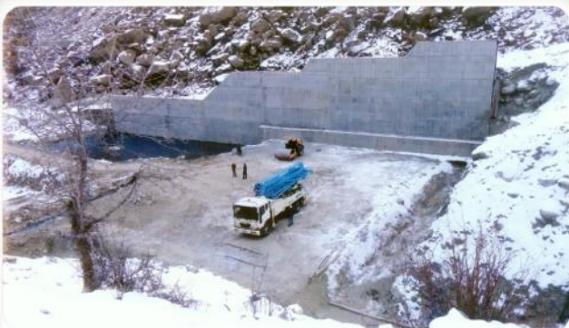
Compaction Work of Stilling Basin
