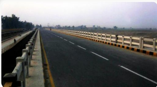
Bridge Over Bhimber Nullah on Old G.T. Road, Gujrat
