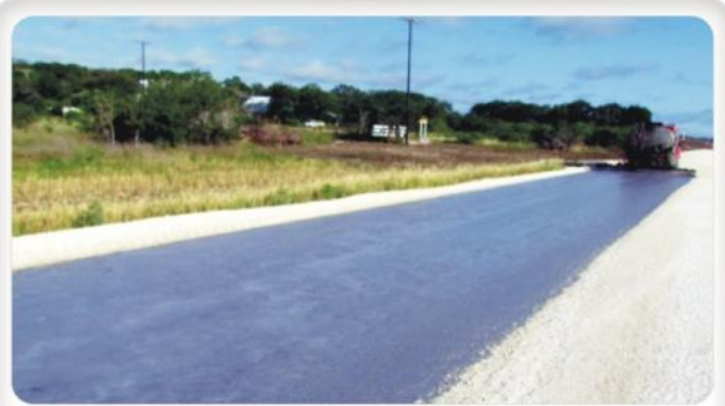
Prime Coat / Tack Coat Activity using Bitumen Distributor
