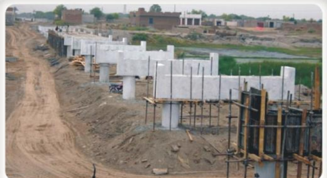
Bridge Structure in Depression Portion for Sullage Carrier Works
