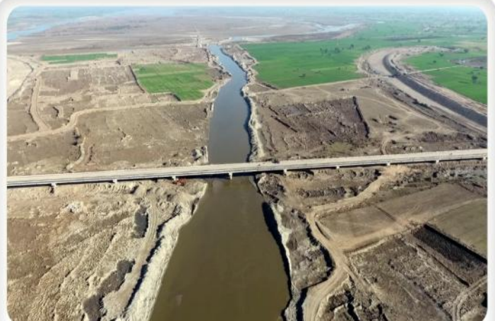
An aerial view of Completed Bridge over River Jhelum at Langarwala Pattan District Sagodha.
