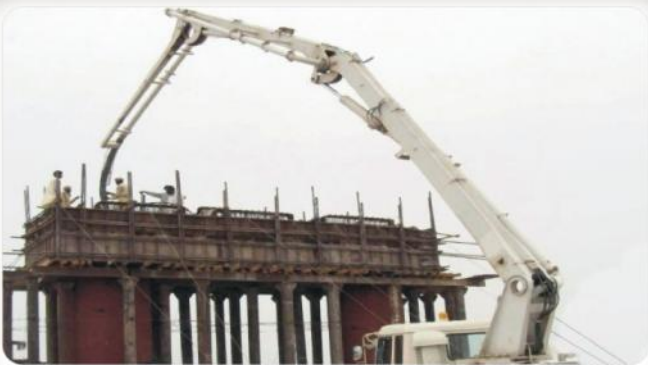
Concrete Pouring in Pier Transom through Concrete Pump
