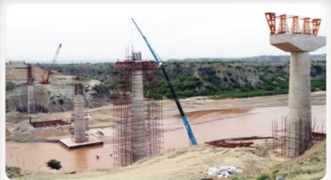
Pier Column Construction Activity Column Height upto 103 feet
