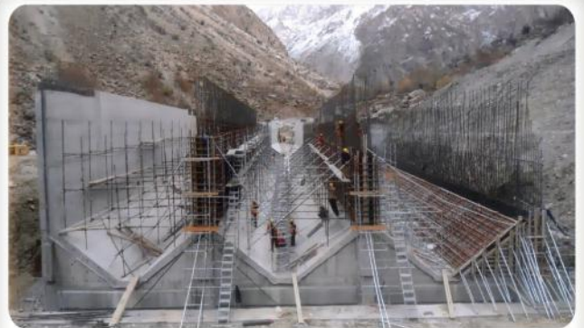
Formwork of Sand Trap
