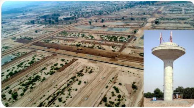
Infrastructure Development Works at Sector-H, DHA, Multan.
