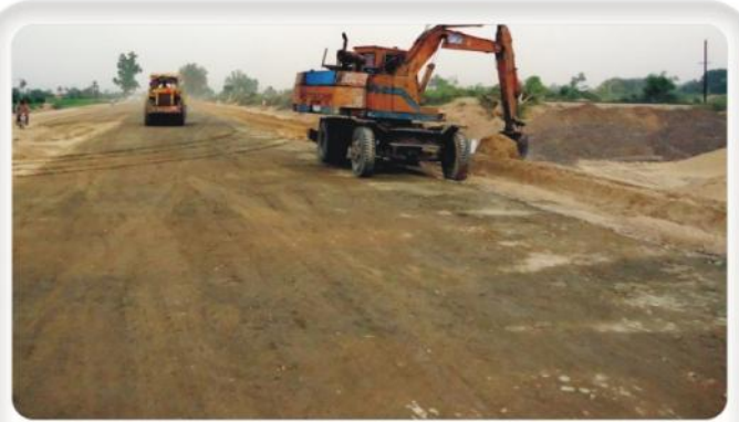
Compaction of WBM Base Course & Preparation of Earthen Shoulders
