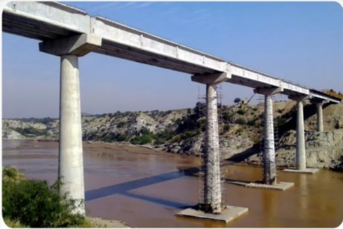
A View of Completed Structure of High Level Bridge over River Sowan, District Attock
