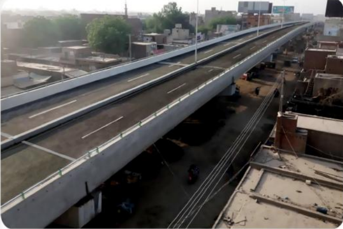
A top view of Completed Bridge Structure Depalpur Chowk Flyover, Okara.
