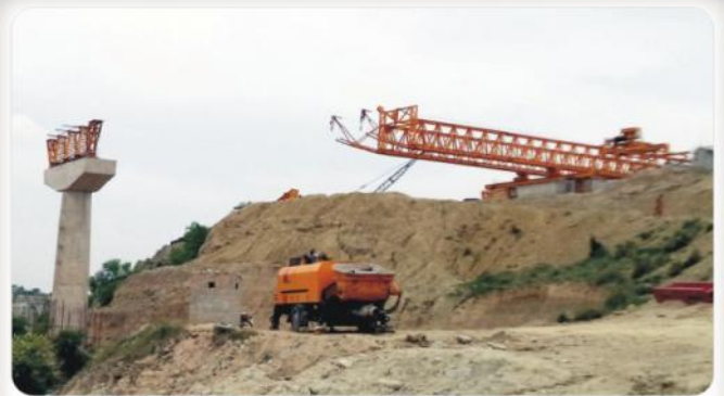
Launching of Concrete Girder using Trussed Type Launcher
