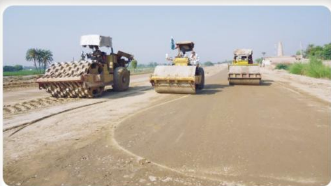
Sub Base Course Activity Compaction using Vibratory Roller
