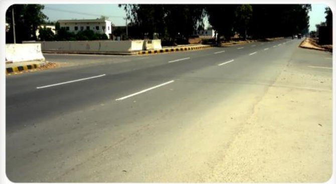
Construction of Additional Lanes along both sides of R.B Canal, Faisalabad
