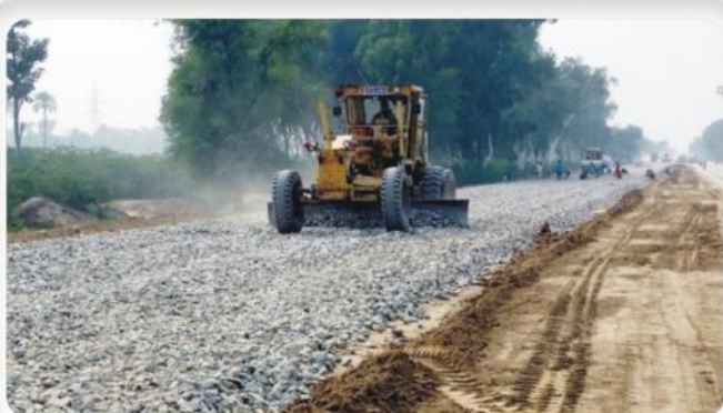
Leveling of WBM Base Course Using Motor Grader
