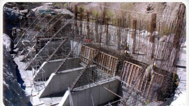
1st Wet Soil Structure (Formwork of Wall)
