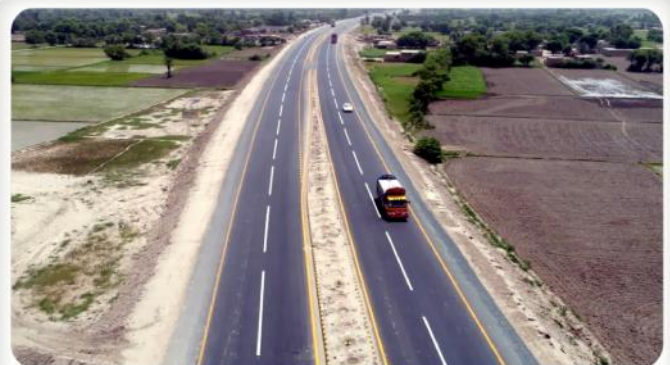
An Aerial View of DCW Muzaffargarh - D.G. Khan Road
